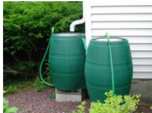
Two rain barrels in sequence capture water off a roof about 19x12 feet in size, providing a ready water source for lawn and garden. Photo courtesy of the University of Rhode Island Cooperative Extension Healthy Landscapes Program.
